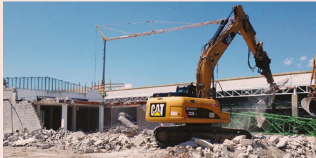
Demolition of old premises
